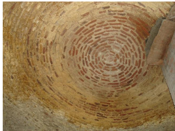
Figure 5 Traditional roof construction of one of the
