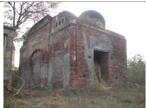
Figure 15: Mosque is being used for storage purpose.
