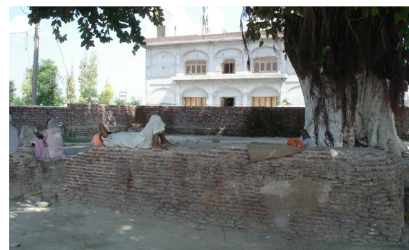
Figure 19: Remains of a historic wall
